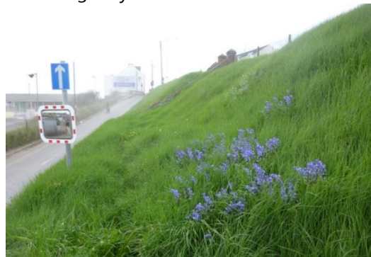
Basin Road North embankment
