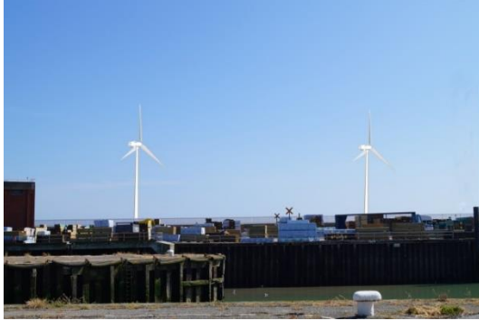
Wind turbines at Outer Layby
