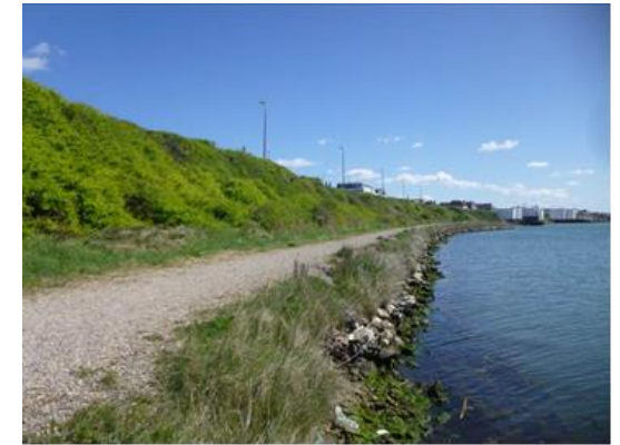
North Canal Bank
